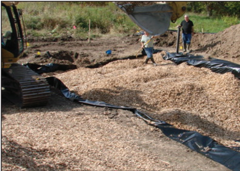
Wood chips being placed in the bioreactor chamber.
